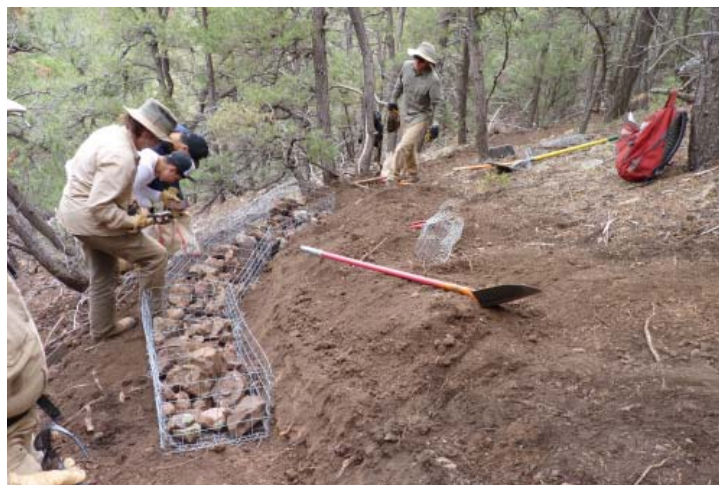
Reineke Construction crew members and volunteers reinforcing switchbacks on the north side of the La Piedra Trail. July 2013
